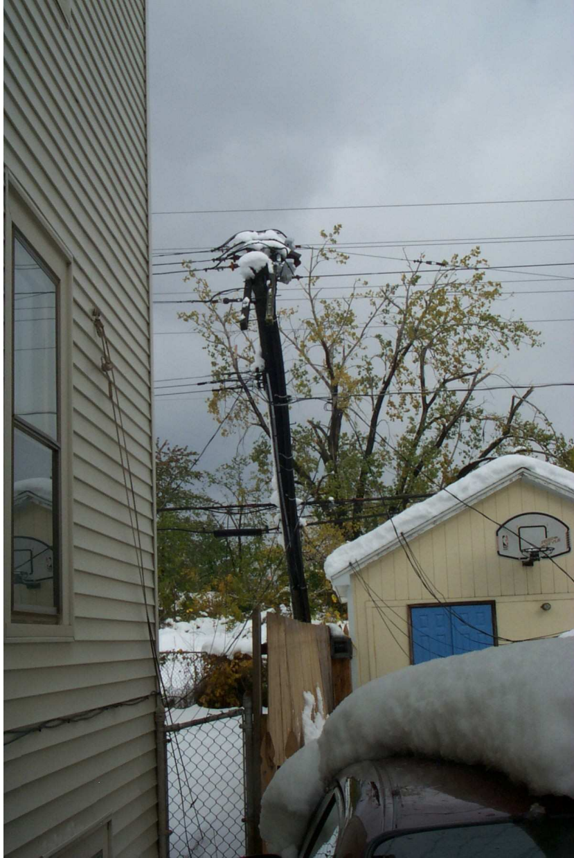
Figure 26: Utility Pole Tipped Over
